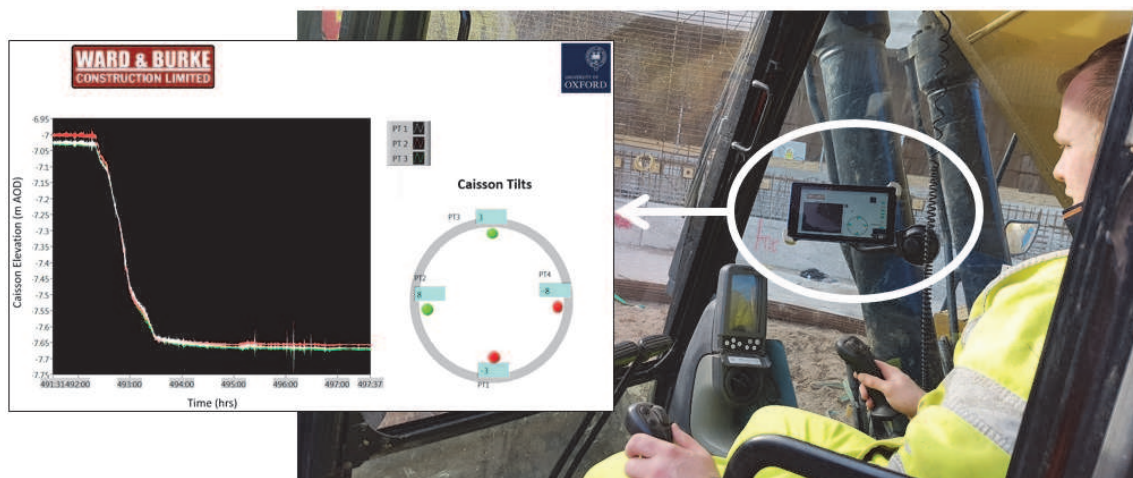
Fig. 4: Monitoring dashboard located in excavator during caisson sinking
