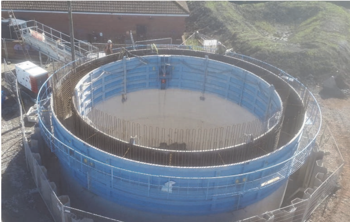
Fig. 1: Sloway Lane caisson under construction
